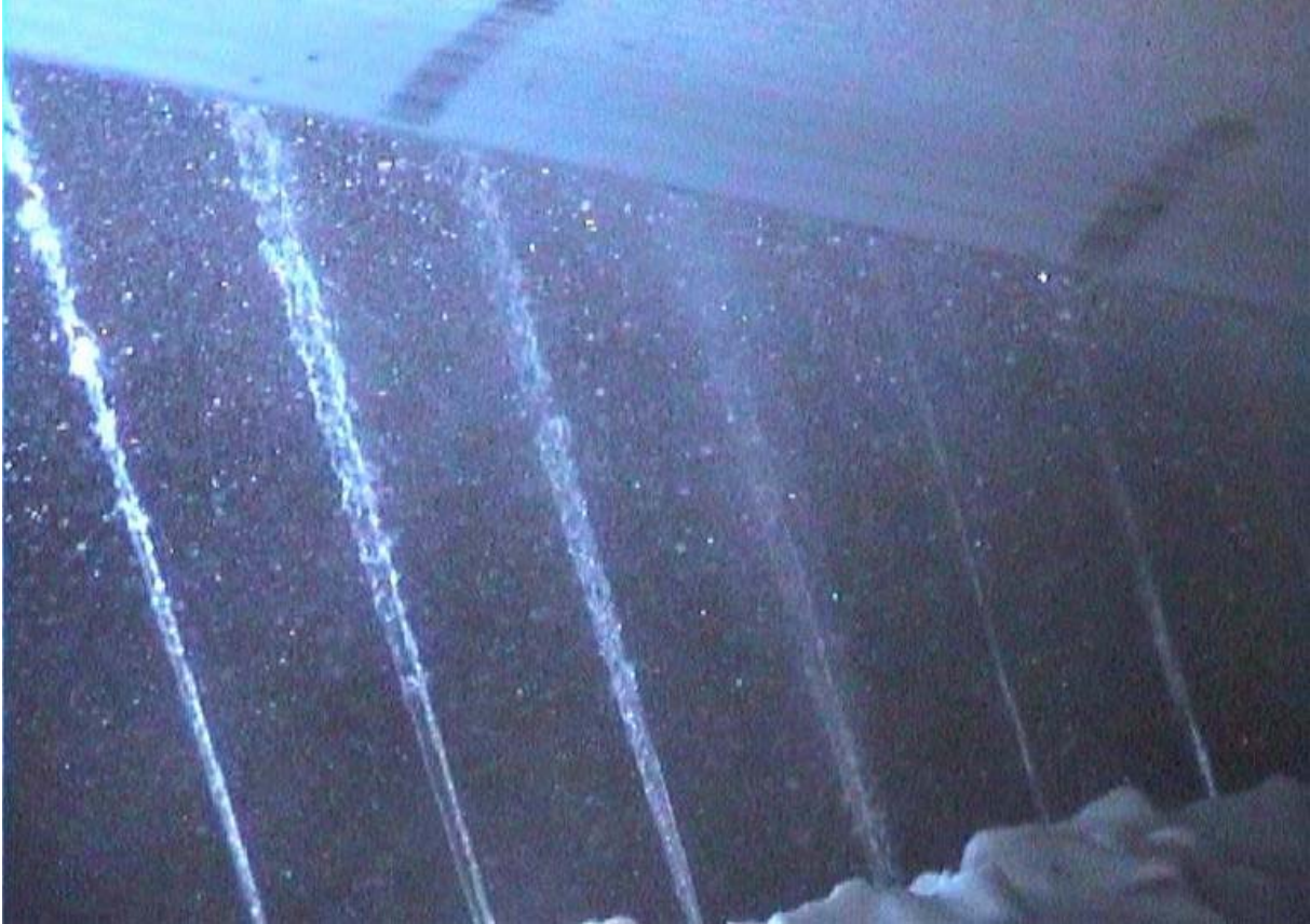
Picture 13: Poor jet quality resulting from nozzle wear by cleaning brush
